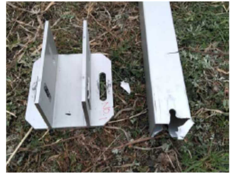
図Ⅲ-2-(ロ)-(i)-D-16 柱材下縁端部せん断力破壊
