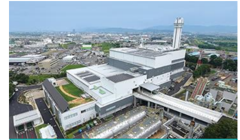
Energy from Waste Plant
