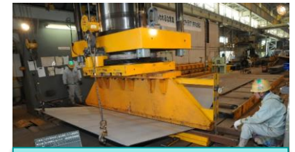
Bending steel plates
