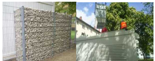
Figure 6 Installation of noise insulation equipment and silencers outside the Energy Center
