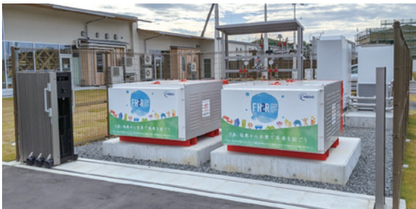
Fuel cell batteries provided to roadside market in Namie Town. Stationary fuel cell batteries use hydrogen to generate power used for electricity and heat in public facilities.
