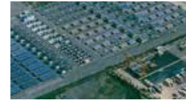
1986 Experiments on a large-scale grid-connected photovoltaic power system started for the first time on Rokko Island in Hyogo Prefecture
