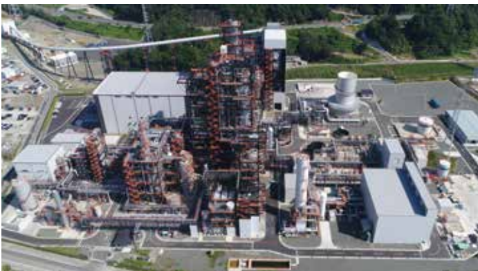
Nakoso IGCC power plant
