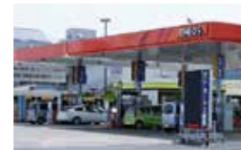
2012 Commercial model demonstration hydrogen station constructed
