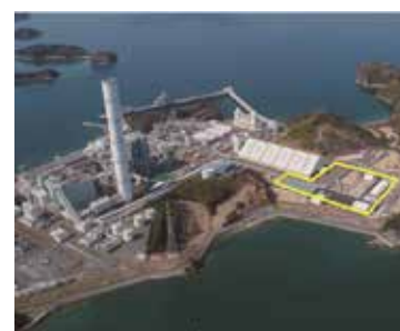
R&D and Demonstration Base for Carbon Recycling
