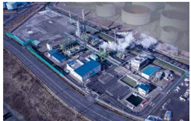
Tomakomai CCS Demonstration Center
