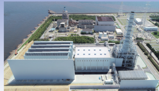
T-point 2, combined cycle power plant at Takasago Machinery Works, which is in operation (Photo provided by Mitsubishi Heavy Industries, Ltd.)
