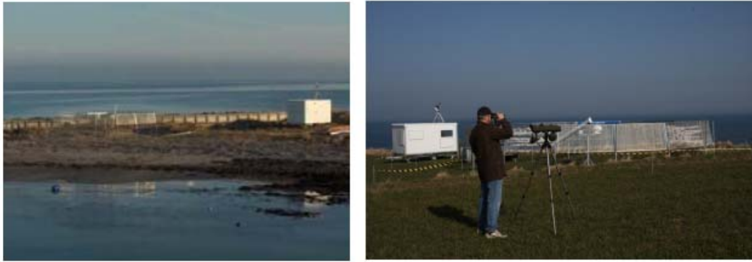
Figure 3-11 The radar installation at Anholt Harbour and Gjerrild Klint
