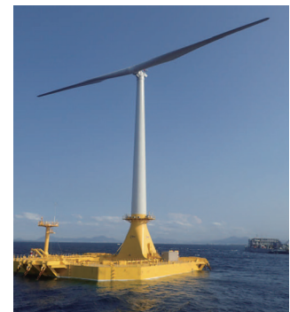
Completed barge-type floating offshore wind turbine for demonstrations
