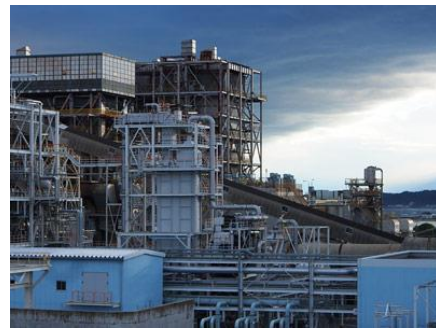
Nakoso Power Plant No. 10 unit of Joban Joint Power Company achieved a new world record for IGCC continuous operation.
