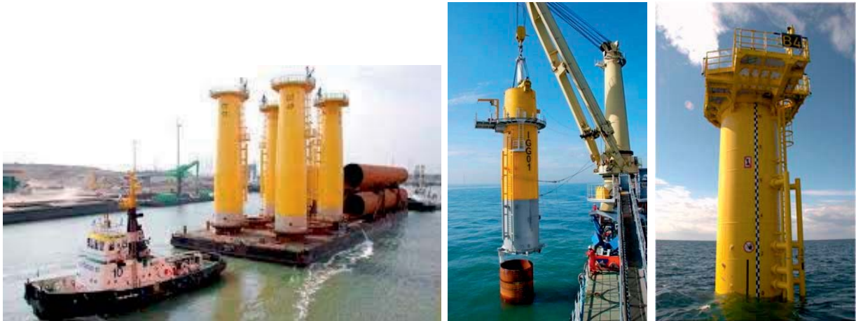
左図・中図:heavyliftspecialist com.、右図: Ballast Nedam(2011)
