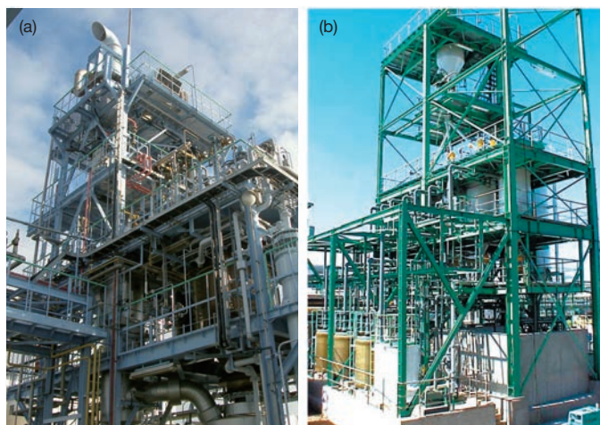
Figure 1 Fluorinated Gas Disposal Facilities Using Submerged Combustion Method
