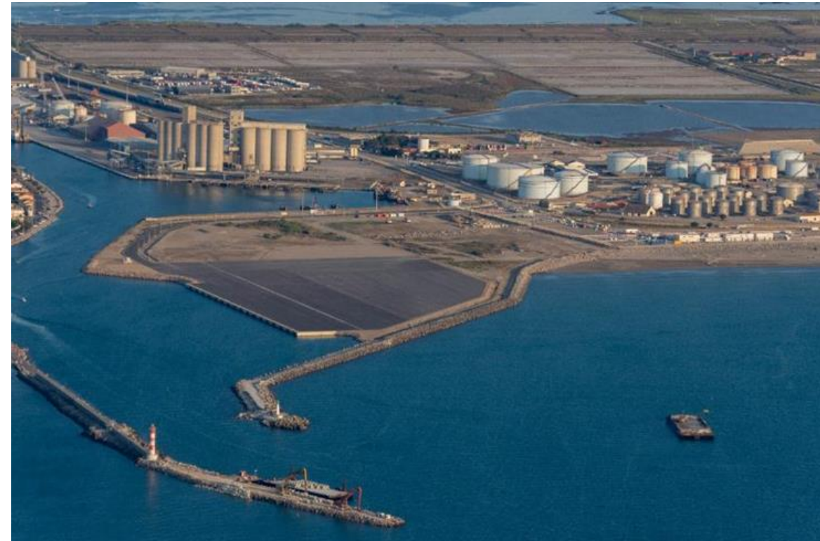
Heavy load quay - August 2021
