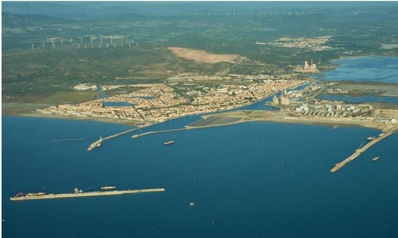
Breakwaters works - August 2021
