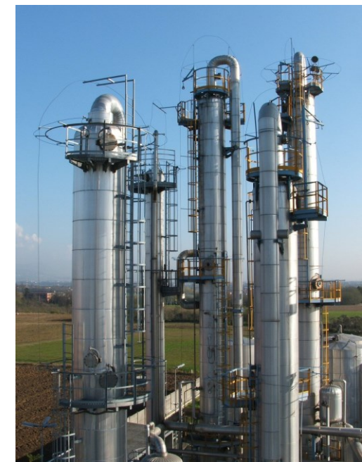
A double effect distillation plant, Wikipedia commons, CC 3.0
