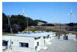
Wind turbine generator
